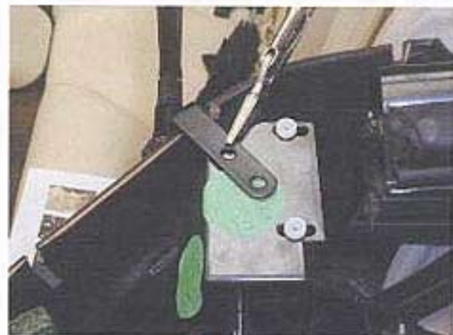
Fig:6 View showing placement of passenger's side larger piece of angle iron prior to drilling.
