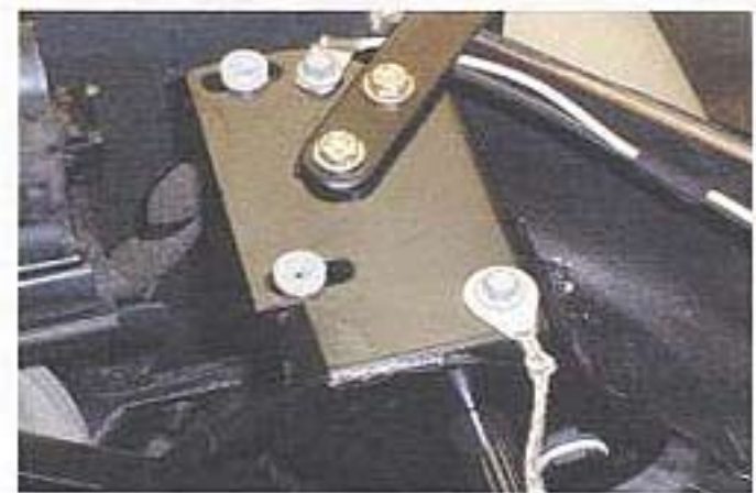
Fig:3 Showing larger piece of angle iron correctly bolted to steel plate by 6 mm bolts and nuts (underside) (Driver's side)
